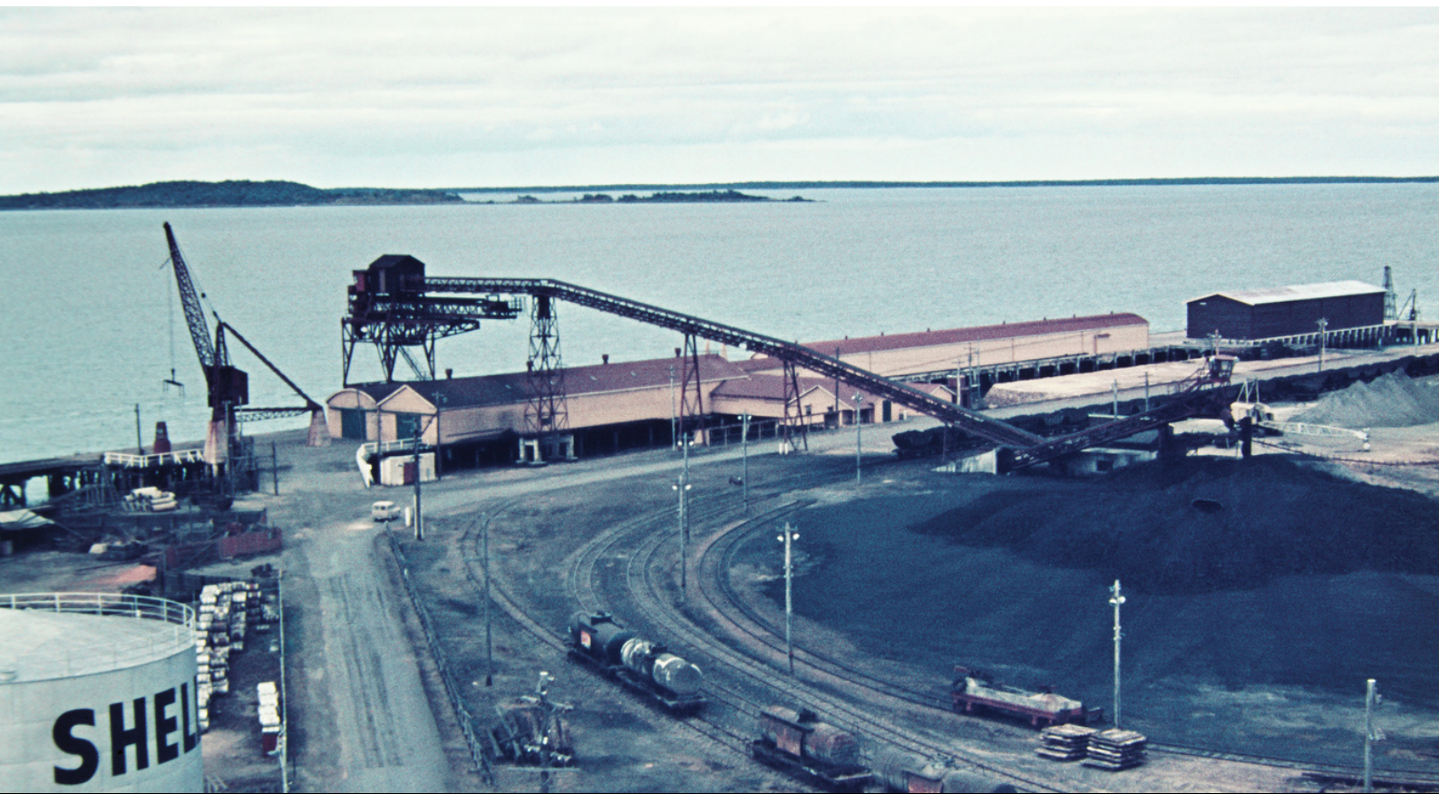
The Port of Gladstone, Queensland, May 1957. Photo: Queensland University of Technology.
